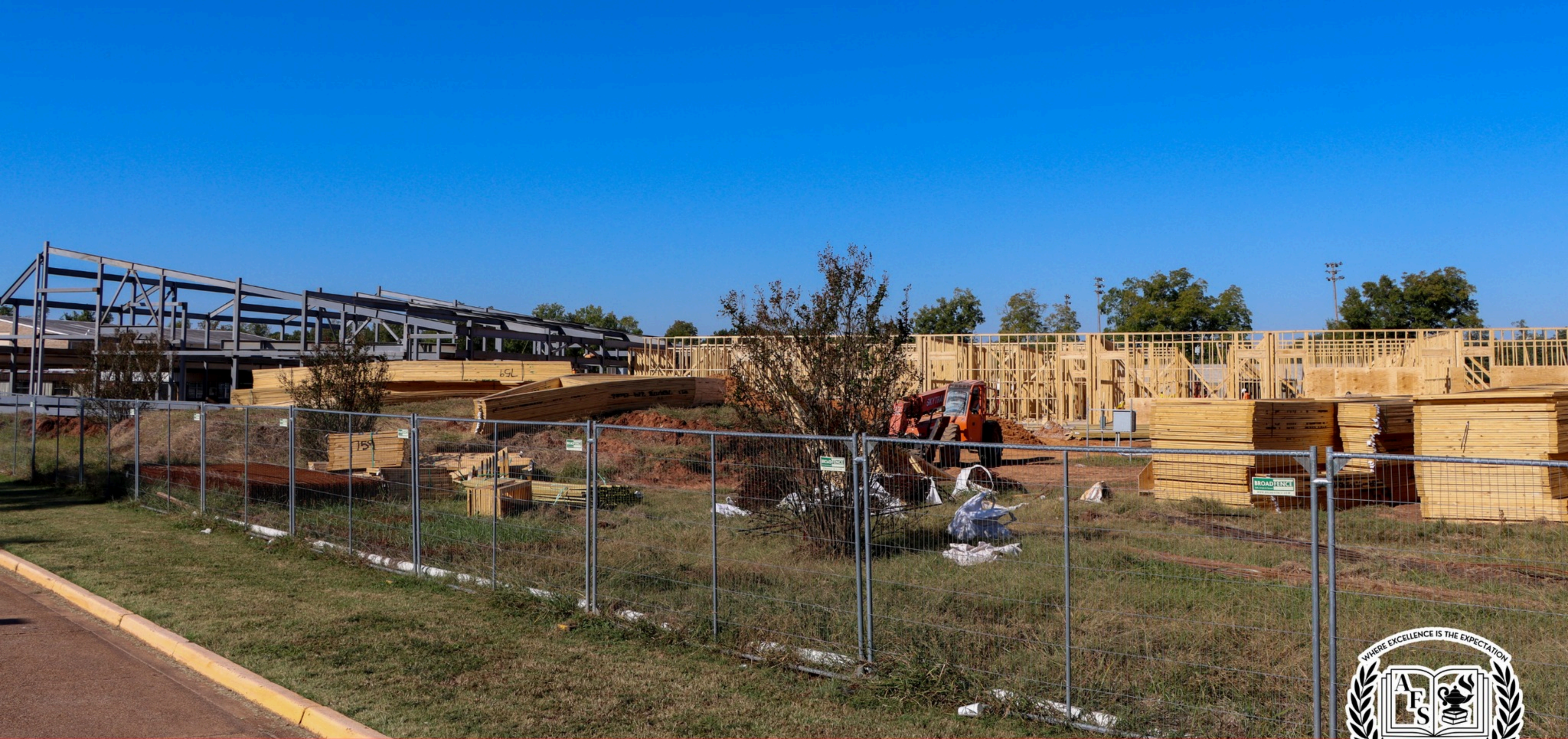
Arthur F. Smith Middle Magnet New Building Construction
